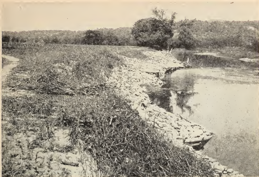
FIGURE 9.—Streambank protected by stone-filled log-crib jetties (wing cribs) supplemented by stone riprap.
